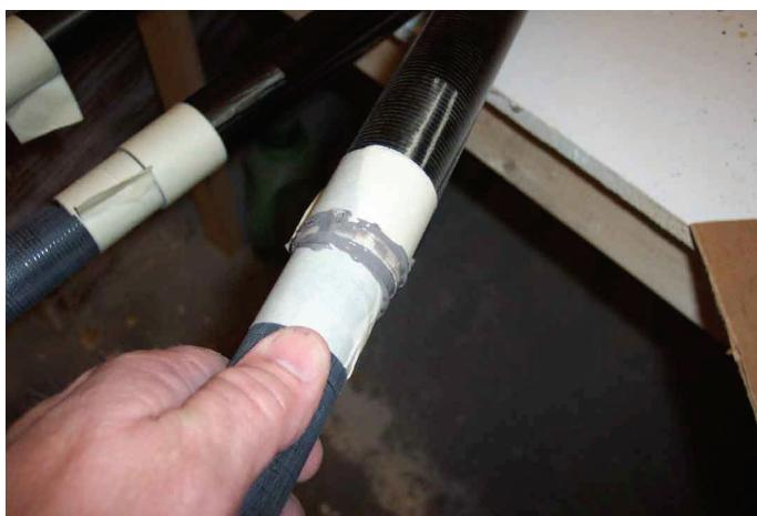
Take a paper towel and wipe the excess JBW off the tape and set it aside. I like to set mine so this will hang over the edge of the bench or where ever the work space. Do the rest like the first.
