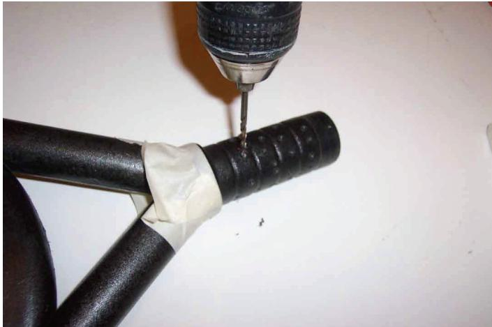
Now to prep the Foot and the pointed End Cap. To prep this and the point, take a small drill and just drill the surface that gets inserted into the pole section to dimple sized dots..I use a 3/16" drill bit. This will create small little areas that with the JB Weld cured will help keep you from pulling the point or foot off when you stick the pole in the mud...again, trust me on this one.
